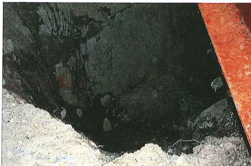
CK2231 Left Abutment (2)
