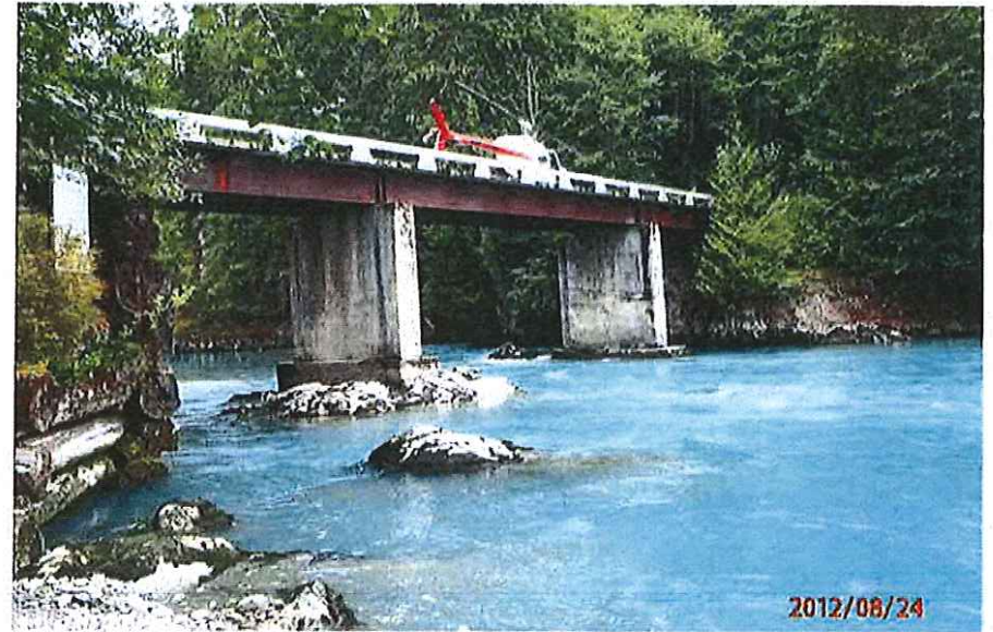
CK2231 From Downstream
