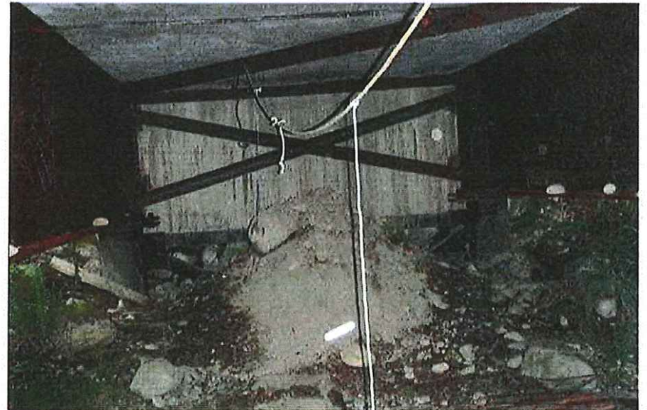
CK2231 Right Abutment (2)
