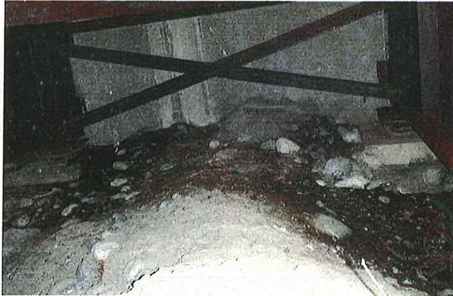
CK2231 Left Abutment (3)
