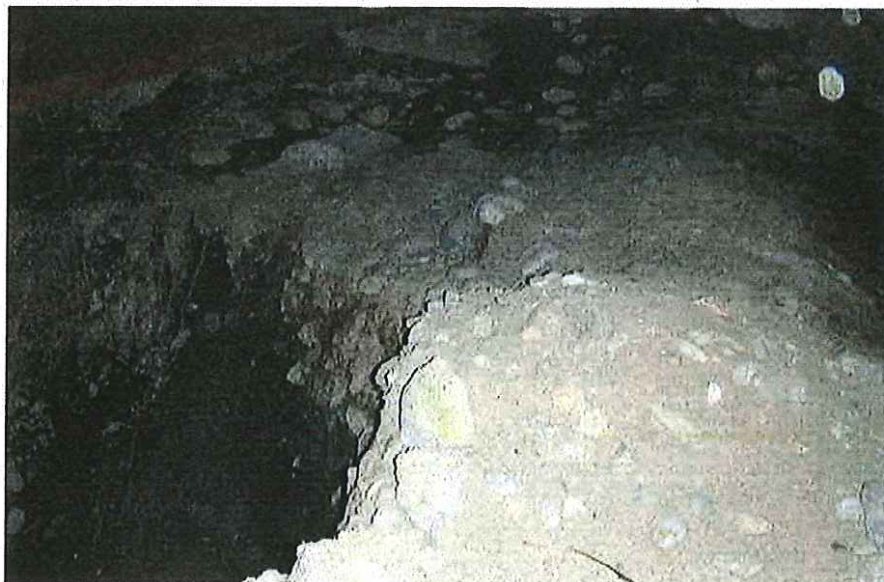
CK2231 Left Abutment (1)
